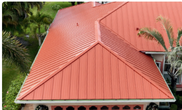
Pictured Top Right and Bottom Right, a roof with no sign of oil canning
