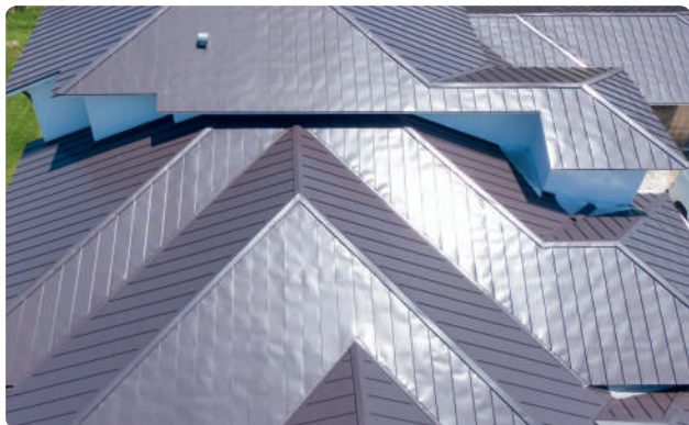
Pictured Top Left And Bottom Left, a roof with oil canning
